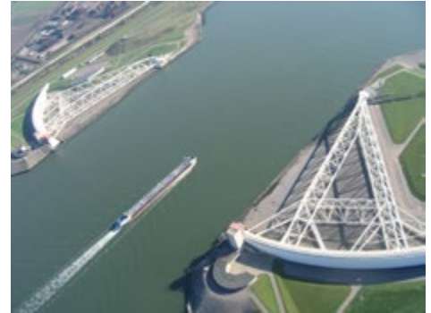
Example of a ship transitioning through Maeslant storm surge barrier gate structures (Photo Credit: John McQuaid)
