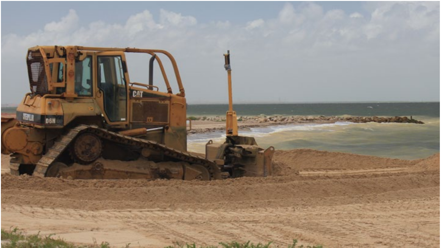
Example of beach renourishment in-progress
